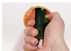
Stripping a cable sheath.
