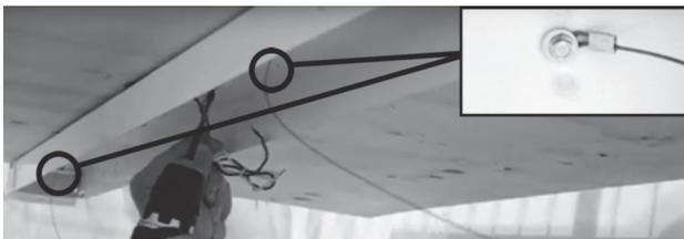
**Note:** To prevent product from falling, secure the retrofit kit to the housing with safety cables.
