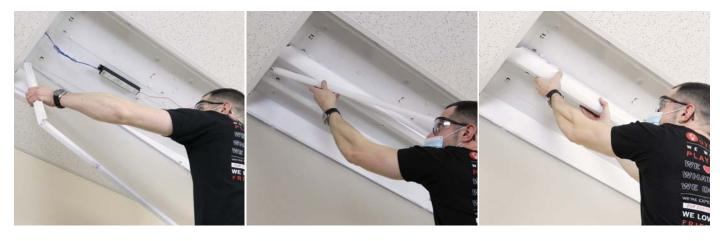
STEP 2 Install retrofit support brackets (x2) and secure with Tek screws. Install optional slide plates, depending on fixture gaps.
