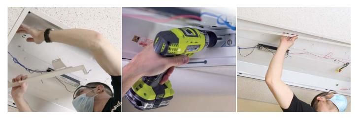
STEP 3 Slide fixture body into keyholes on retrofit brackets. Attach safety cables to existing fixture and apply supplied sticker advising fixture has been modified. Connect input power (including ground) to building wiring. Close panel and secure latches.
